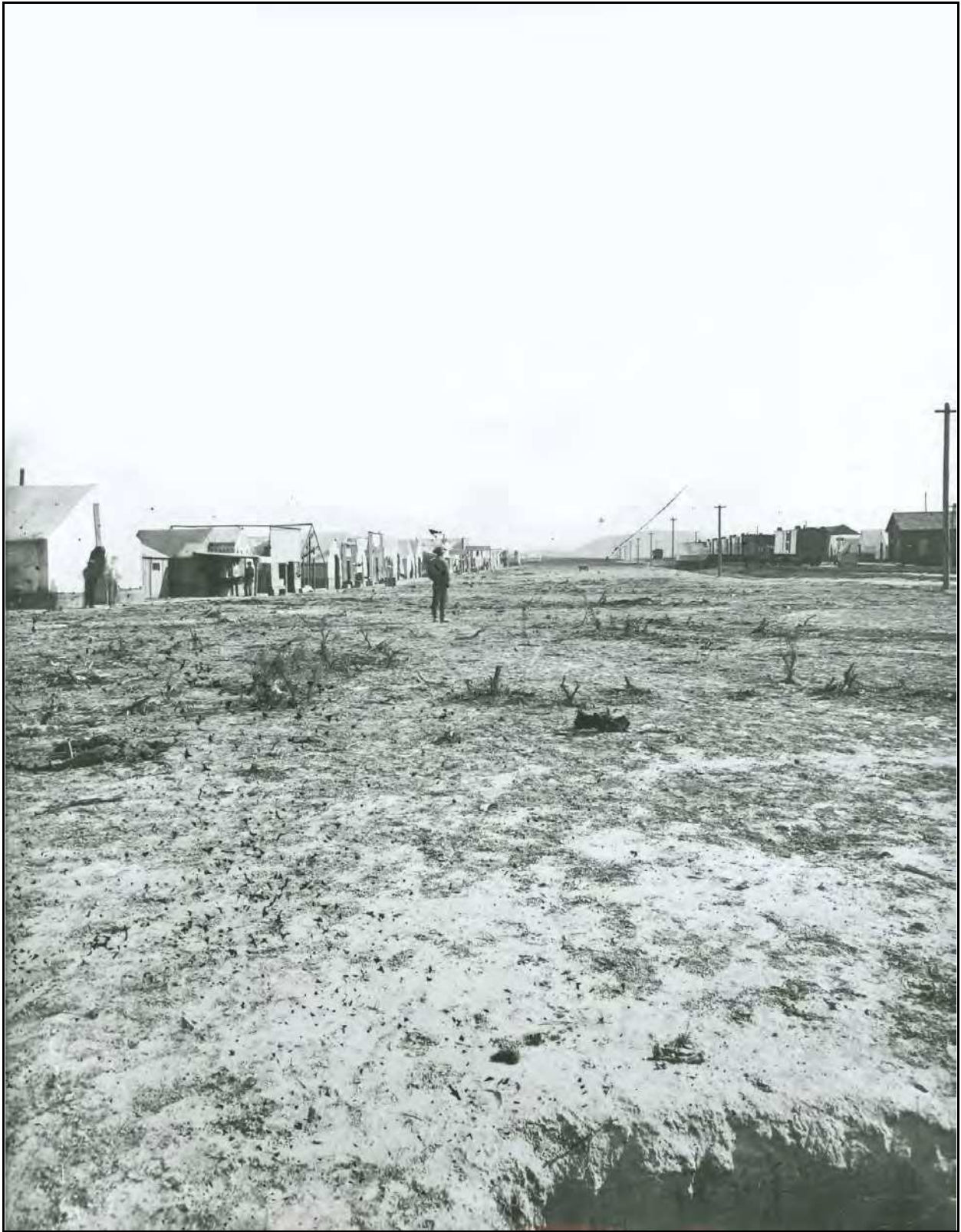
Figure 8.2. The Last Spike Site Looking West, Showing Coarsely Constructed Borrow Ditches and a Central Pacific Spur to the North of the Main Tracks. Photograph by A.J. Russell; courtesy of the Oakland Museum of California.
